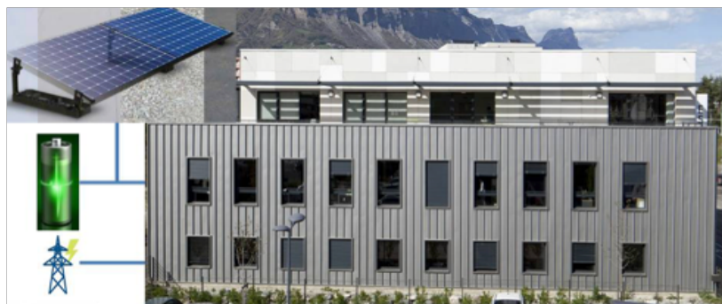
Figure 8-2 Collective PV in Grenoble
